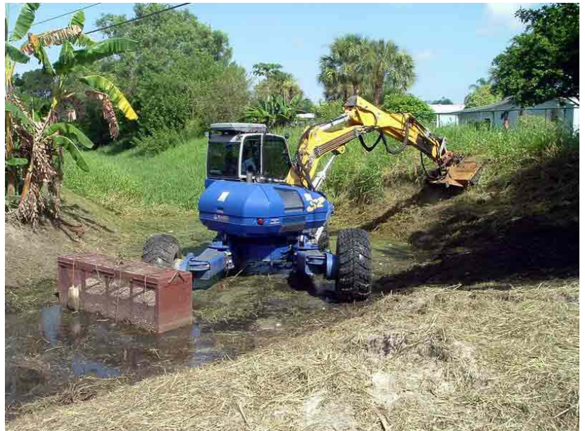
Design: A movable metal box was designed for ease of mobility and mixing of the Floc Logs. Note the Floc Logs placed within the metal box.
