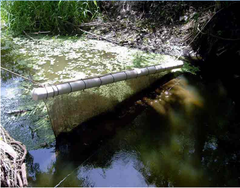
Above: Particle curtain strategically placed to catch the particles that did not settle out by gravity.
